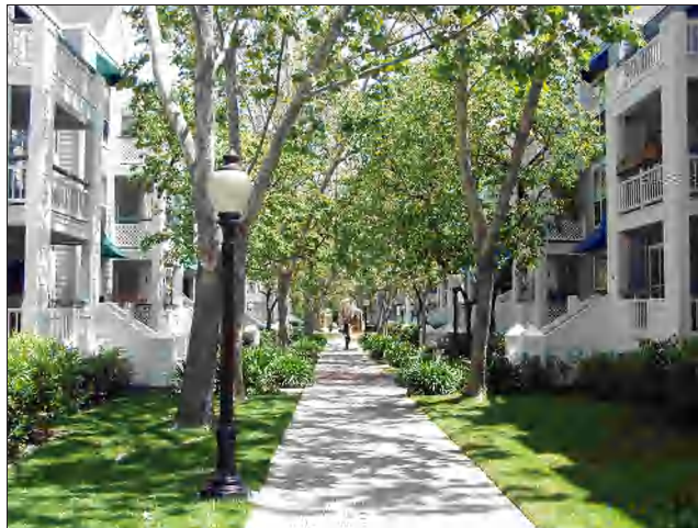
Apartment flats with partially submerged podium parking under individual buildings
