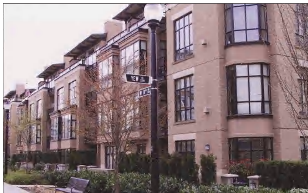
Example of top floor setback and variation in materials and wall planes to break up large building
