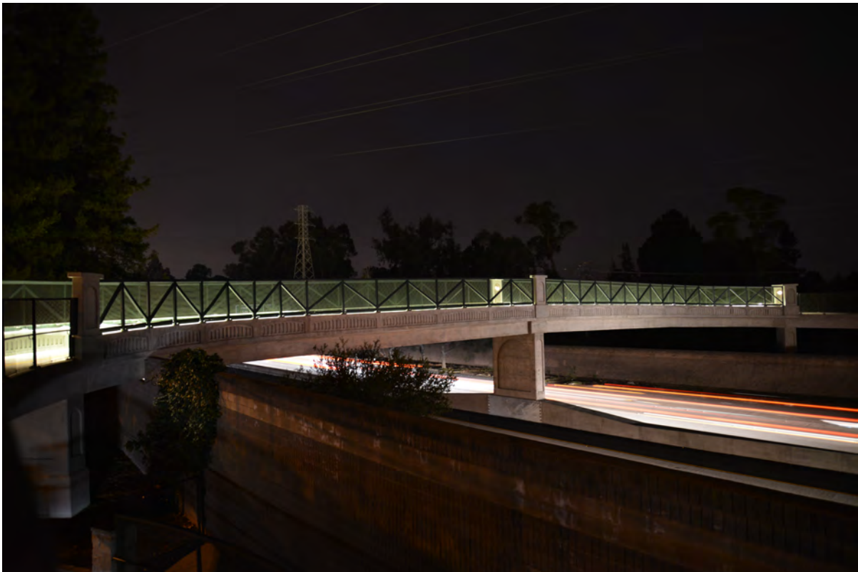
Dale/Heatherstone pedestrian overcrossing spanning State Route 85 on the Stevens Creek Trail.
