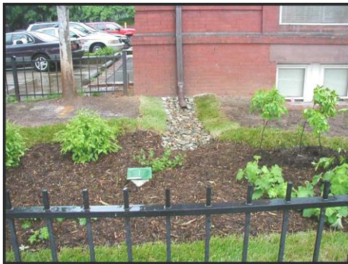
A Low-Impact Development Disconnected Downspout
