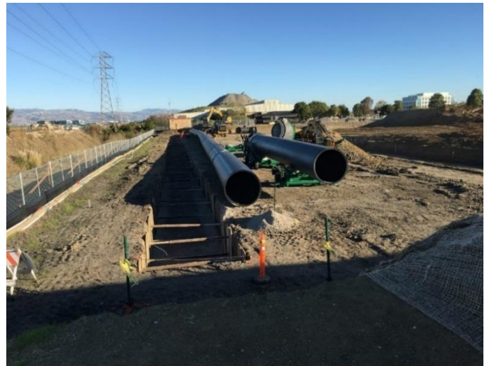
Installation of the primary effluent pipeline.
