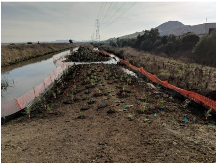
Planting activities in the habitat mitigation area near the Bay Trail.
