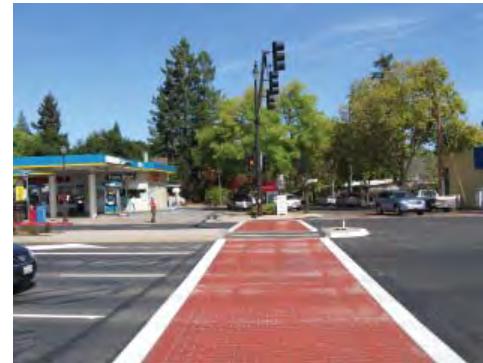
Accent Paving at Crosswalk
