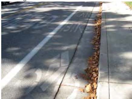
Most streets have dedicated bike lanes, but lanes are frequently narrow or shared with gutter.
