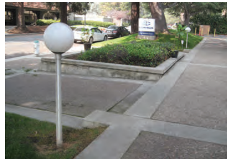
Existing plaza and walkway at Sonora Court
