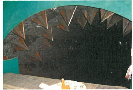
bag-breaker teeth at trommel entrance
