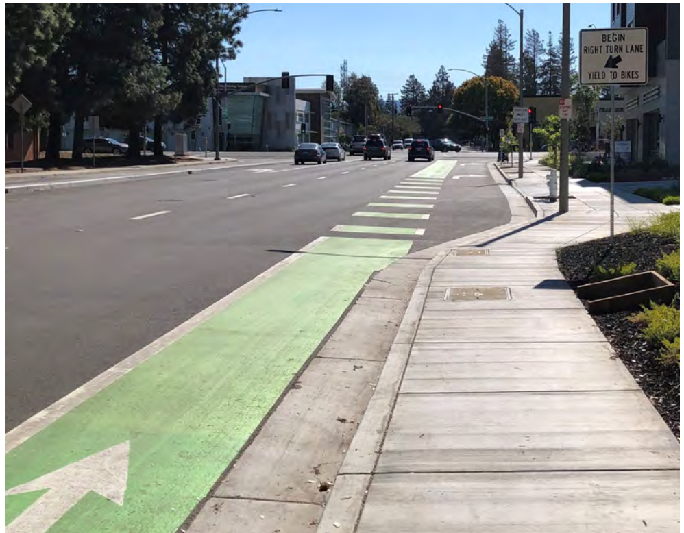
A recent bicycle network improvement on Pastoria Avenue includes signage alerting vehicles to yield.
