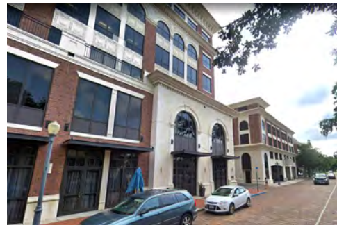
Architectural compatibility between the parking garage (back) and the principal building (front).
