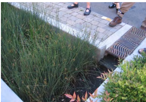
Use of stormwater planters is encouraged to capture and treat stormwater runoff.
