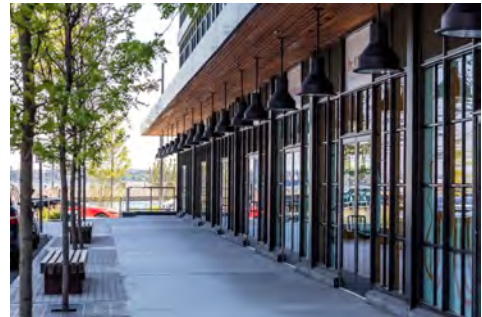
Ground level commercial storefronts should be comprised of mostly transparent windows and doors.
