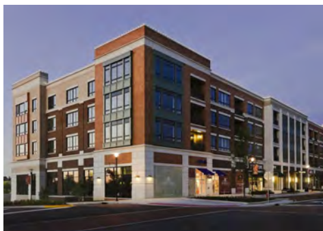
New development incorporating design features that respect the design character of historic Murphy Avenue.
