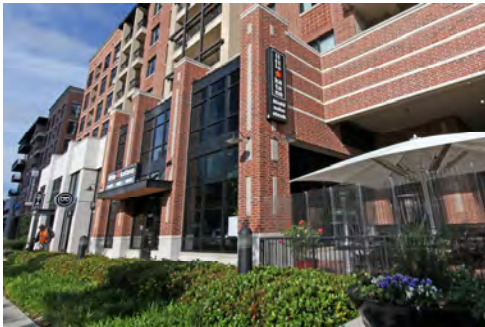
Building set back from the base to provide articulation of the ground floor retail space.
