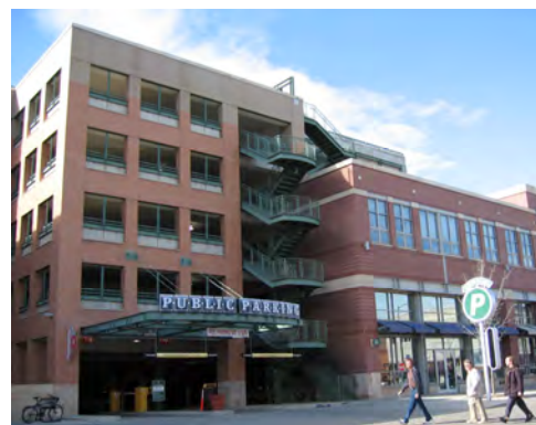
Design stair and elevator cores of a parking structure as key architectural components.
