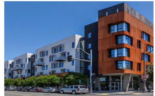
Use of projections and recesses for fenestrations, balconies, and ground floor entries help articulate the building form at the corner.
