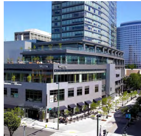
Hotel use with building massing that varies along the length of the block and defines a base, middle, and top.
